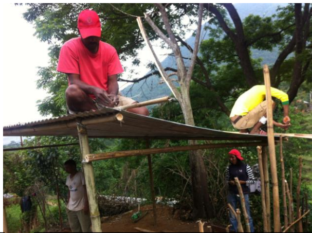
Ramchandra and Rajesh completing the roof of a shed.
