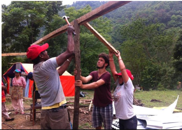
KRMEF Carpenter, our German volunteer Aurel and teacher building a shed.
